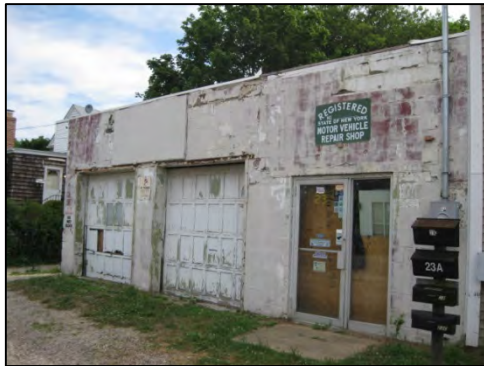
Photograph No. 1: View of vacant building along Railroad Avenue
